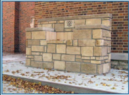
A photo of the outdoor stone fireplace that was constructed next to the west courtyard.
